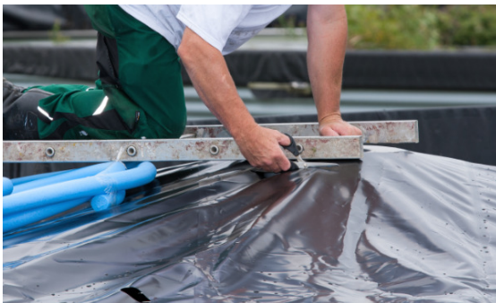
Opening in zeil knippen / cut opening in cover
