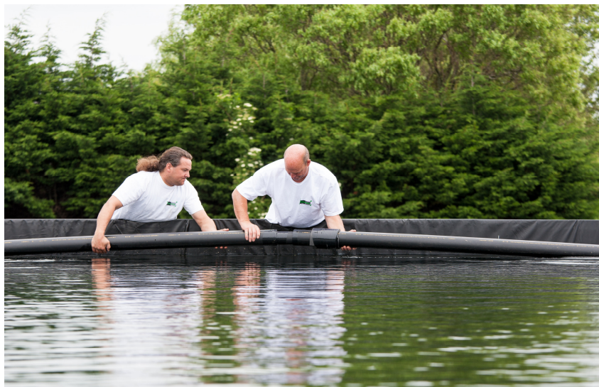
Fig. I circular tube composition consisting of tube; coupling tube; tape and foam rubber
