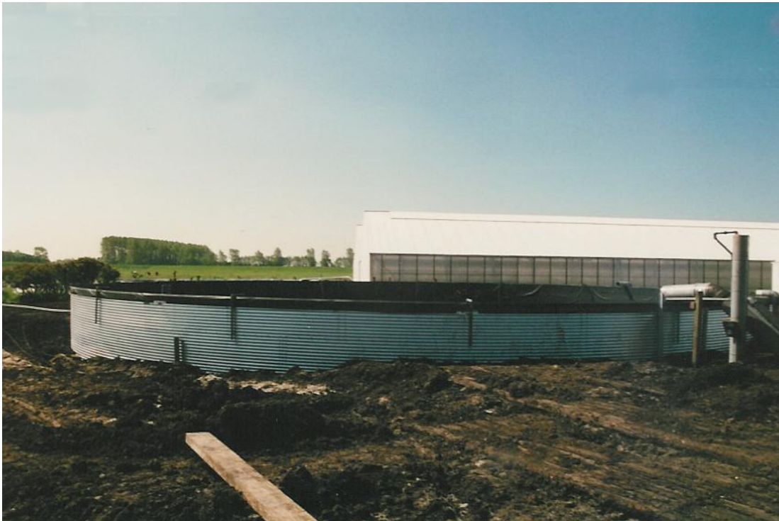
Image 4: end result Aquatex ® EX tankliner Ø 27,31 metres
