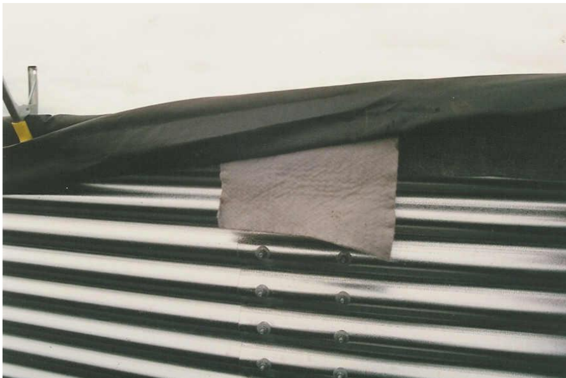
Image 2: bolts and protection sheet
