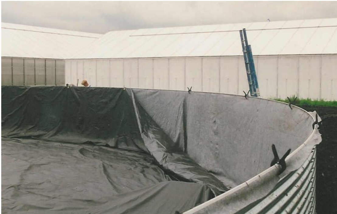
Image 1: attach tank liner and protection sheet to the tank with plastic clamps
